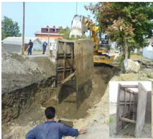
(a) Installation of the initial trench box
