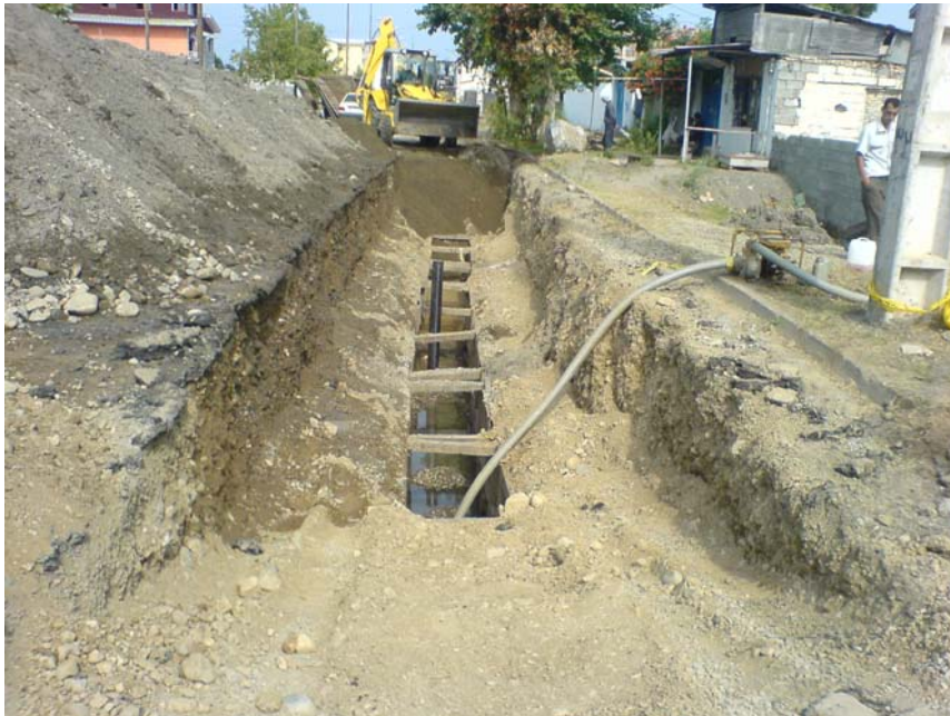
Figure 2: In-trench dewatering of excavated strips a) Installation of the initial trench box
