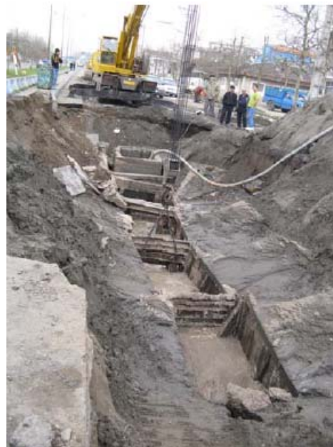
(b) Installed trench boxes
