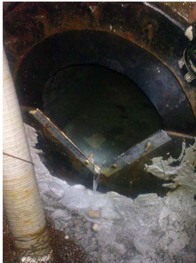
Figure 12: Free weir flow used to measure water leakage
