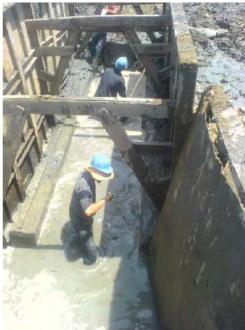
(a) Unstable box wall
