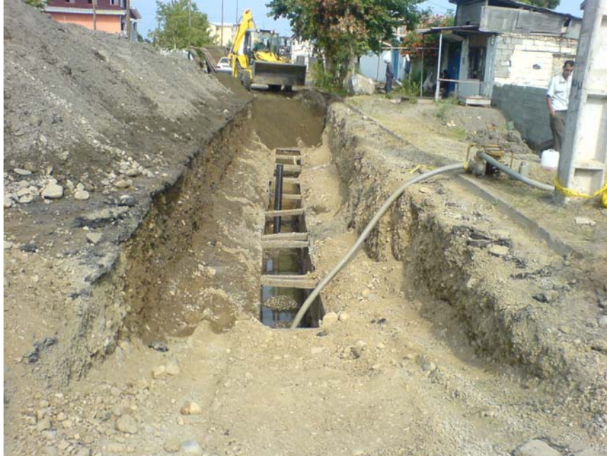
Figure 5: Two-stage excavation method
