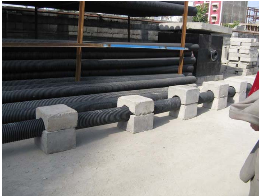
Figure 7: Concrete casings used to protect the pipes against uplift
