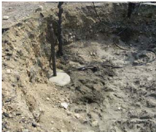
(a) Jet grouting boreholes
